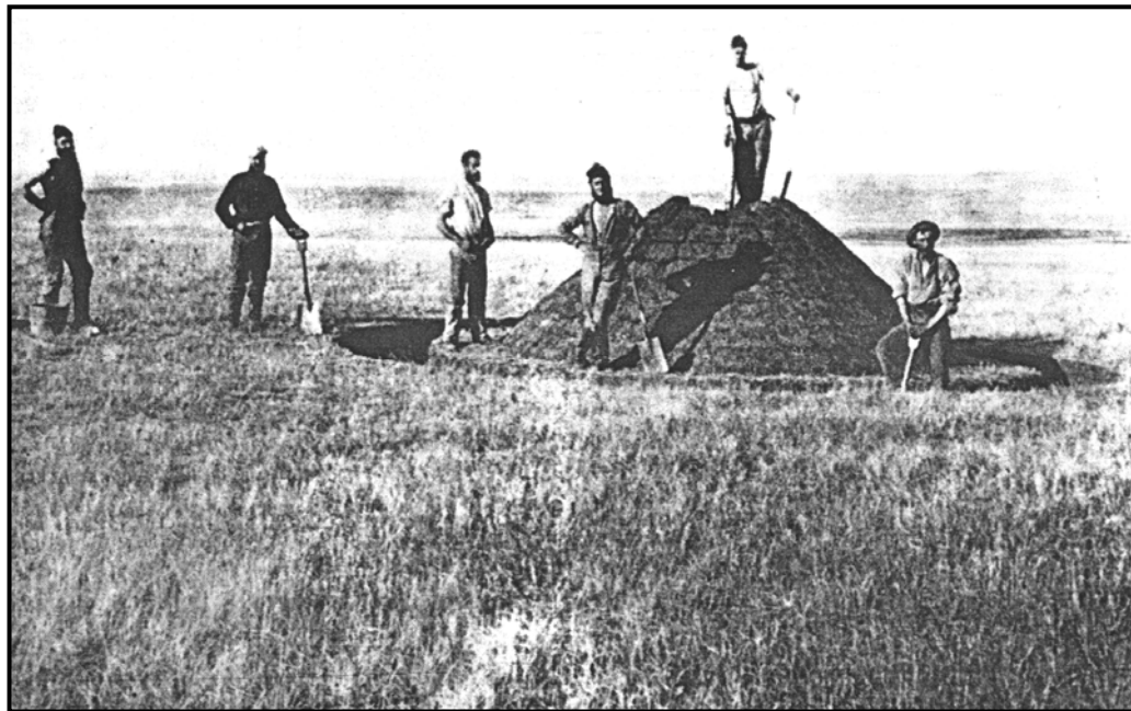
Building a boundary mound at a Section Corner on the U.S.-Canadian border.
